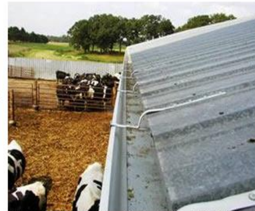
Gutters used to control roof runoff in Benton County, MN. Photo courtesy Benton SWCD.
